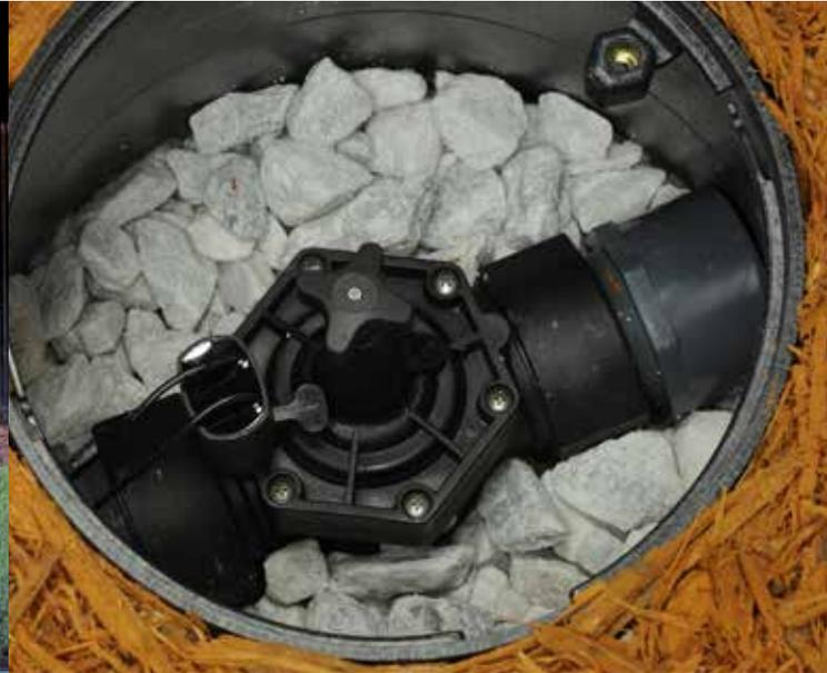
A durable feature-packed electric valve designed to handle irrigation applications up to 200 PSI operating pressure.
